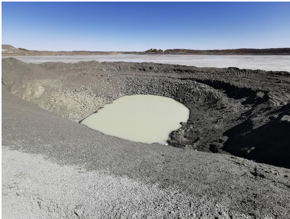
FIGURE 1 VIEW TOWARDS THE INSIDE OF THE “DONUT-SHAPED EMBANKMENT” SEEN FROM THE SOUTHERN DAM WALL CREST. (DATED 12 DECEMBER 2019.)
