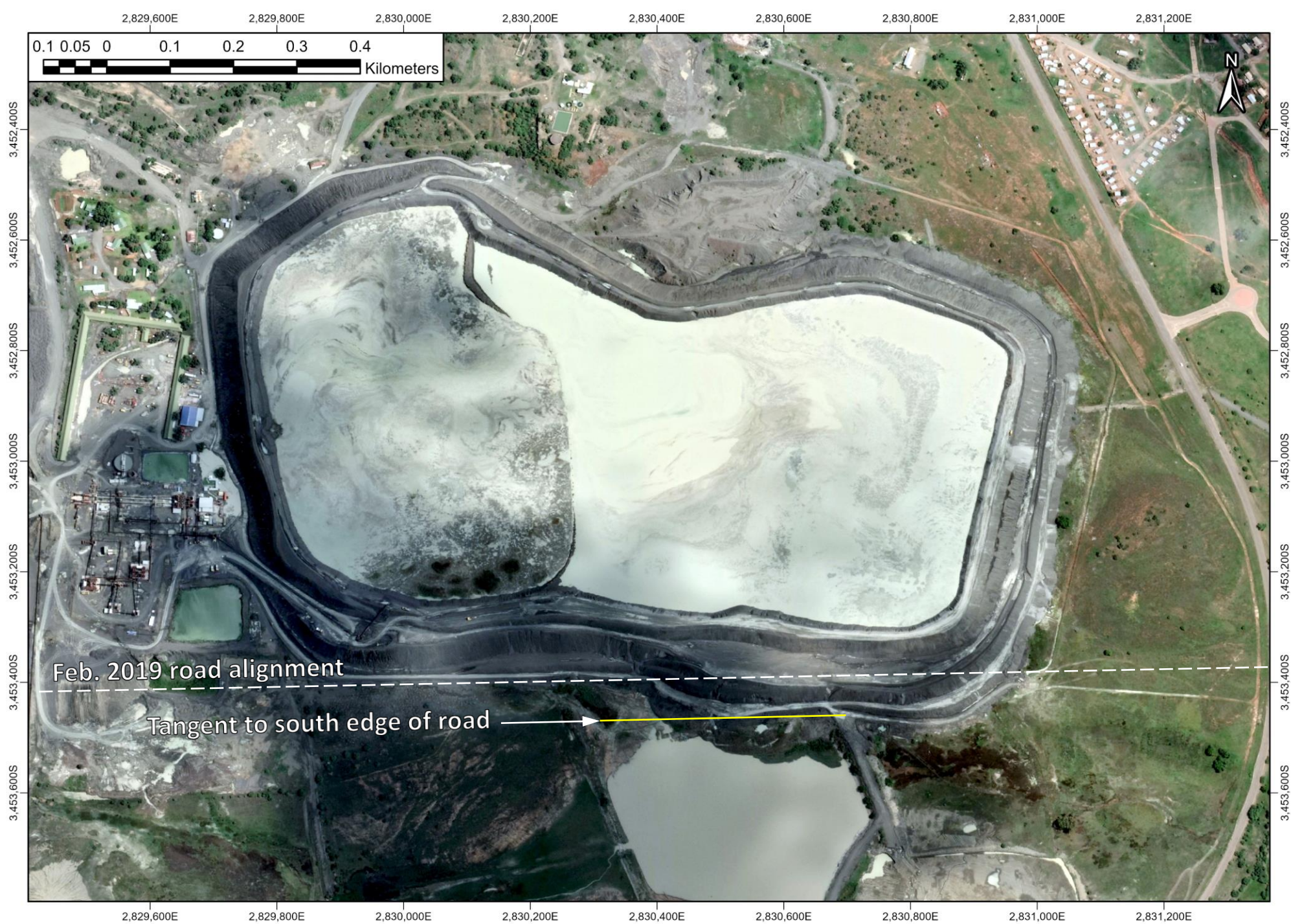
Figure B18: 2021-01-24 WorldView 2 satellite image highlighting the separation between the February 2019 (Figure B10) and the current location of the southern edge of the southern access road.
