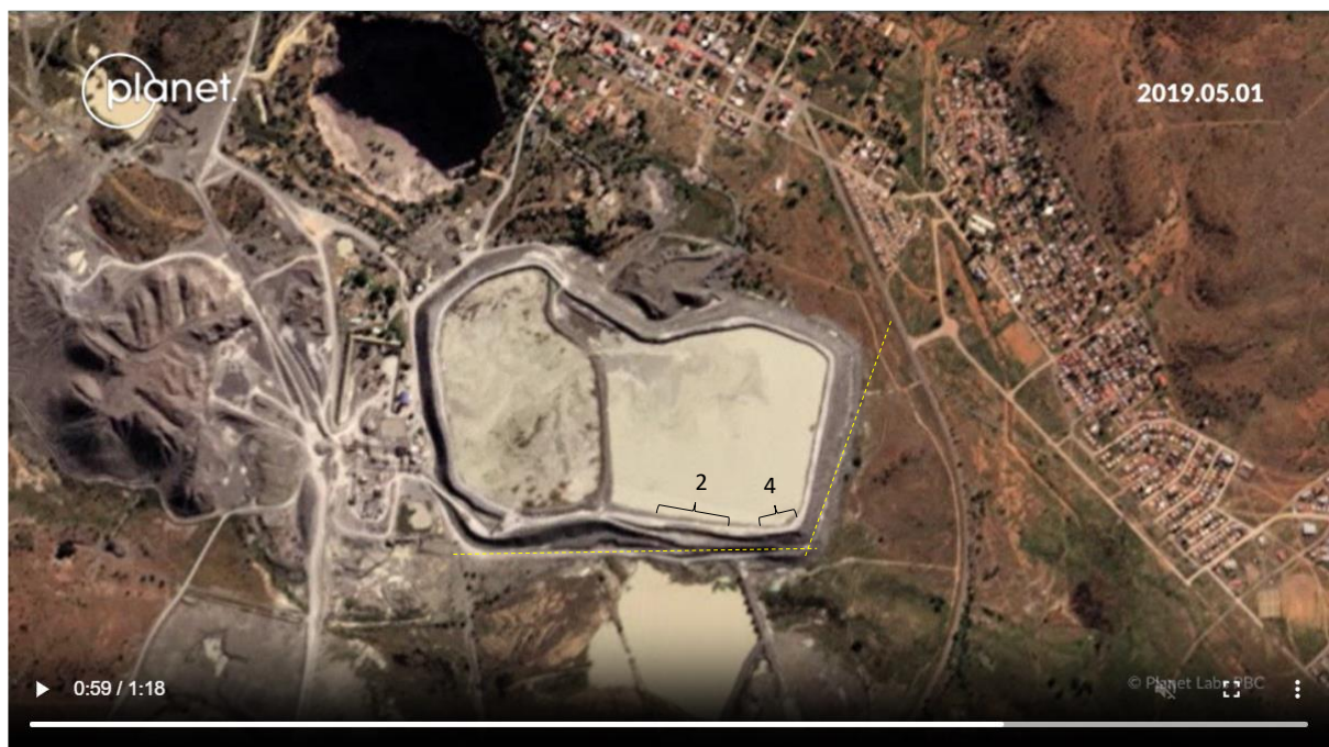
FIGURE 6 PLANETSCOPE SATELLITE IMAGES TAKEN ON 2019/03/30 AND 2019/05/01 SHOWING THE PLACEMENT OF MATERIAL ON THE SLOPE OF THE SOUTHERN WALL OF COMPARTMENT 2.
