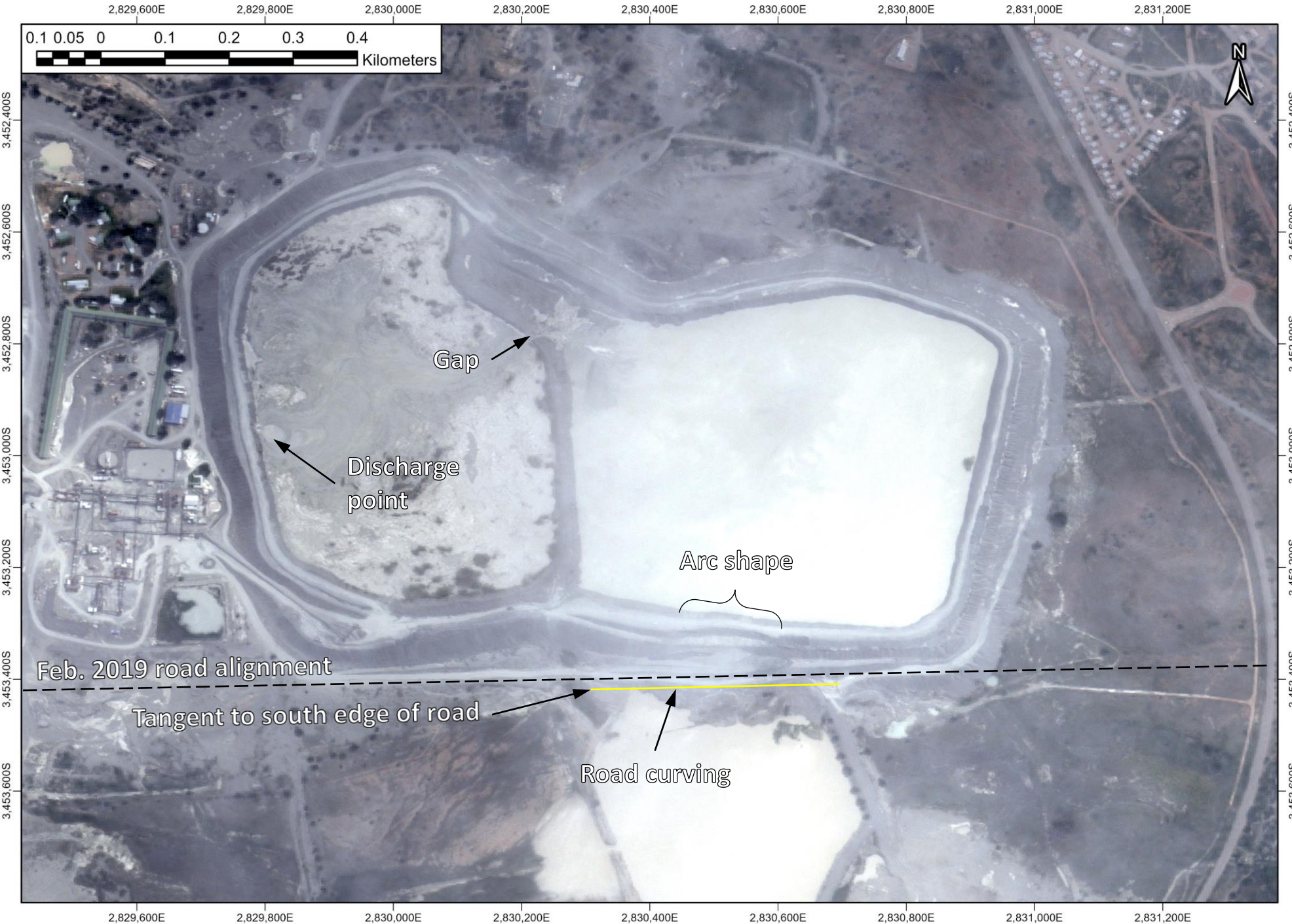
Figure B11: 2019-03-22 TripleSat satellite image highlighting the separation between the February 2019 (Figure B10) and the current location of the southern edge of the southern access road.
