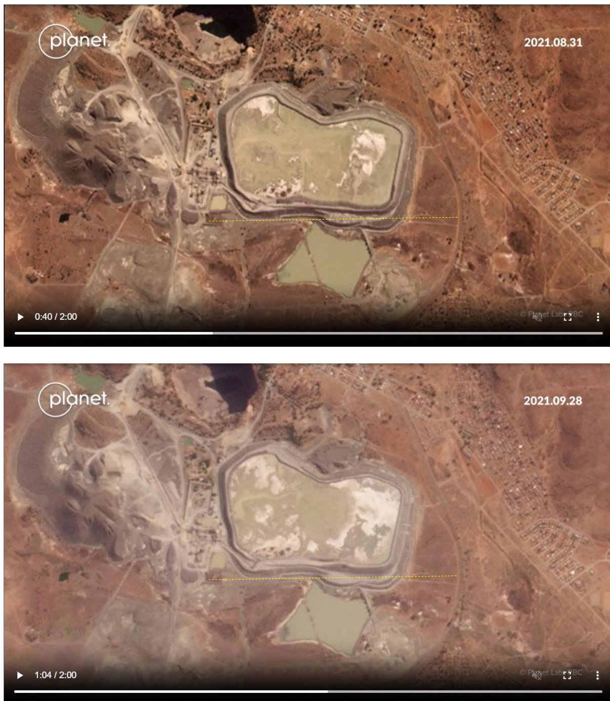
FIGURE 13 PLANETSCOPE IMAGING DATED (A) 2021/08/31 AND (B) 2021/09/28 SHOWING SIGNIFICANT ADDITIONAL DEFORMATION ALONG SOUTHERN AND SOUTHEASTERN TOE OF COMPARTMENT 2.
