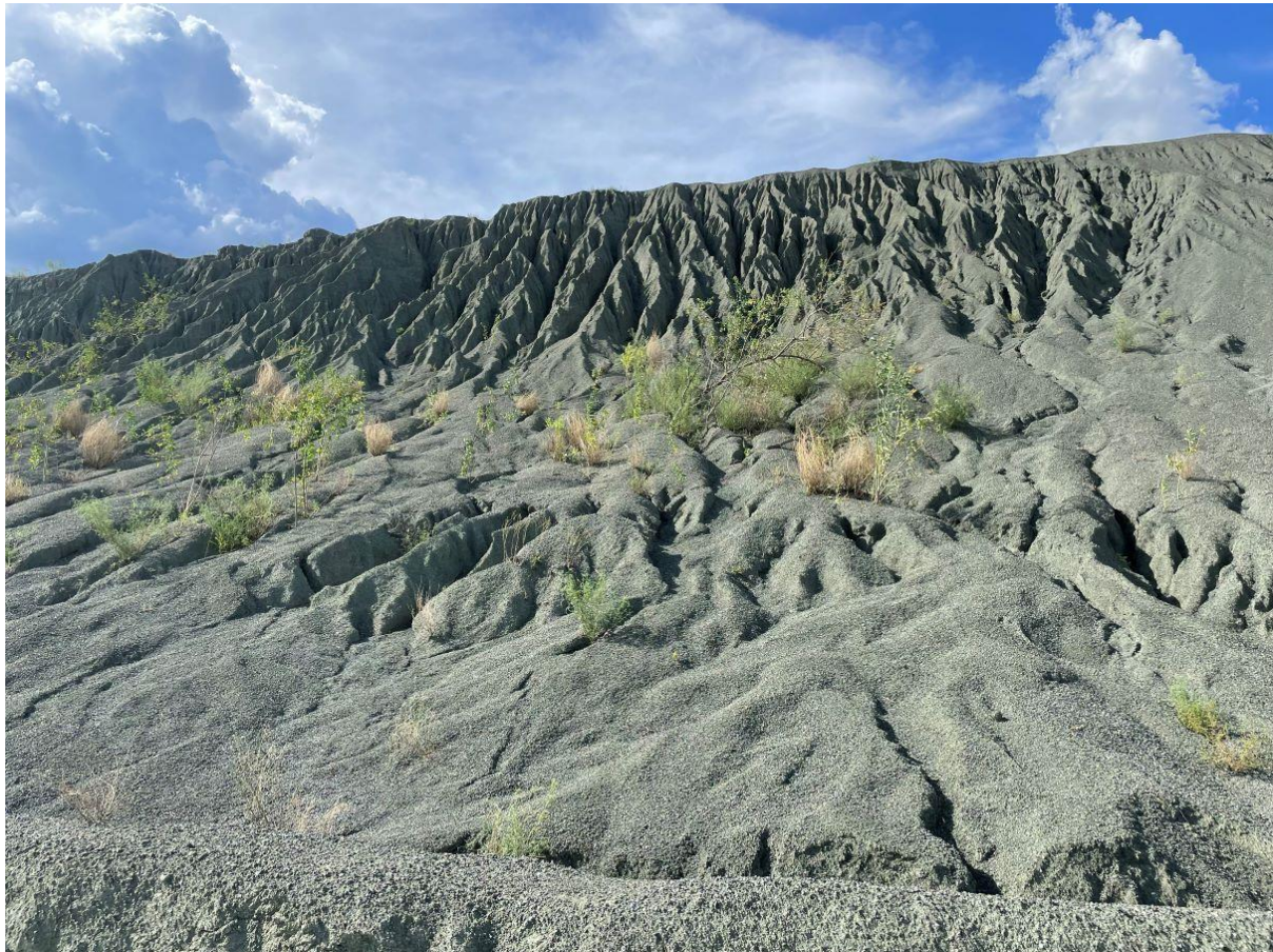
FIGURE 16 SIGNIFICANT SLOPE EROSION SUGGESTION POTENTIAL FOR DISPERSIVENESS.
