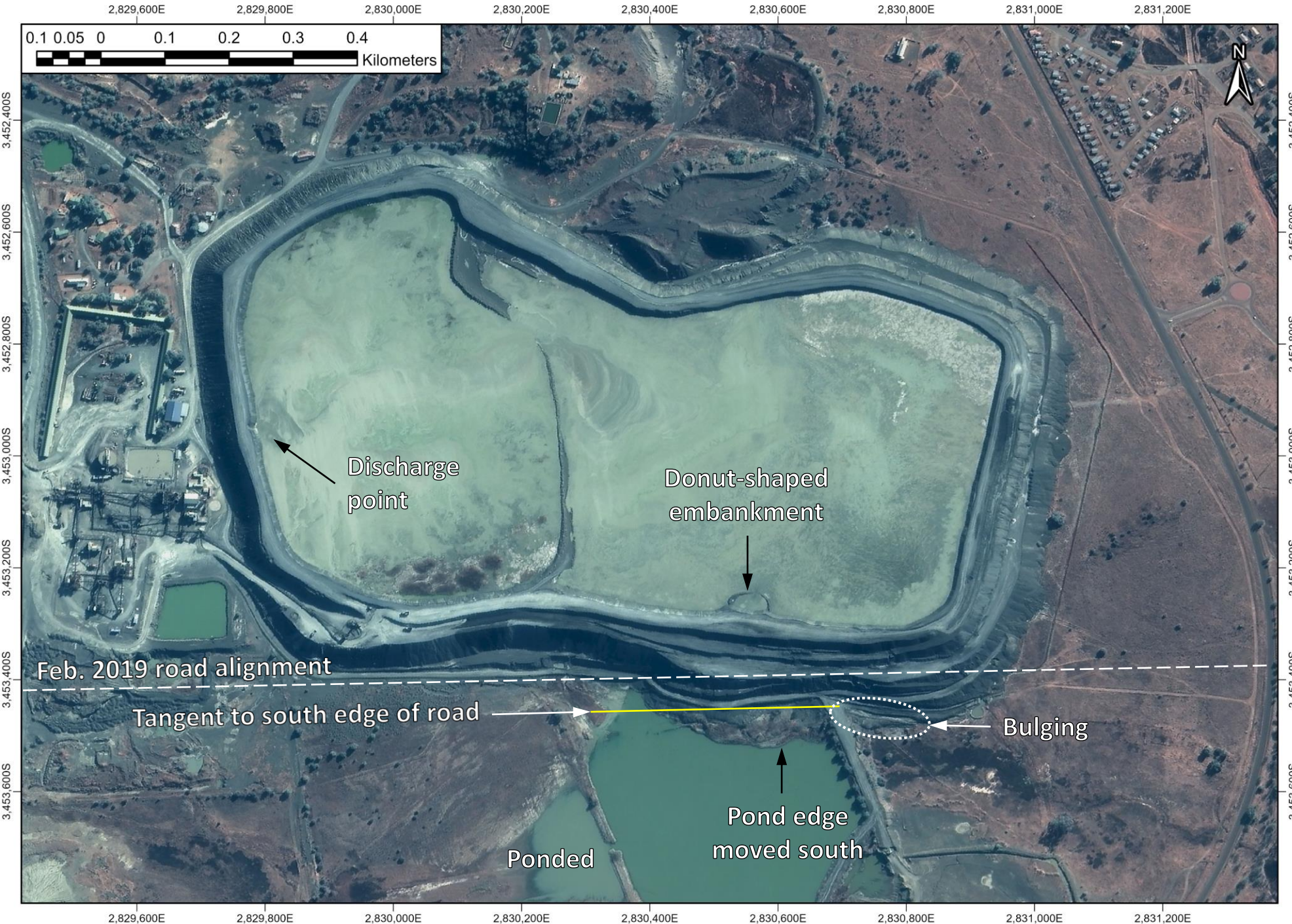
Figure B15: 2020-07-09 Jilin-1 satellite image highlighting the separation between the February 2019 (Figure B10) and the current location of the southern edge of the southern access road. Remnants of the donut-shaped embankment built against the southern wall are visible.
