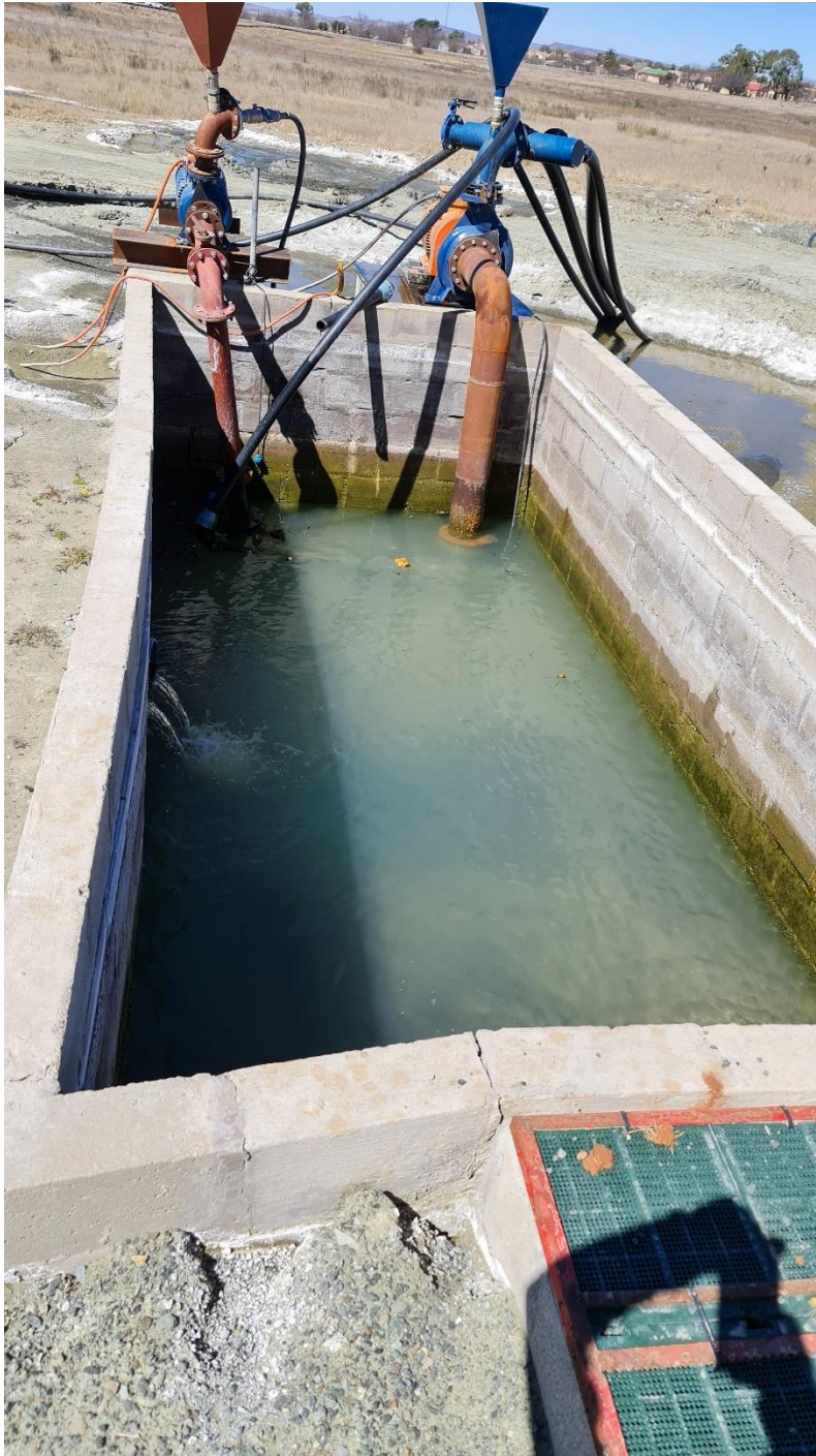
FIGURE 10 CURVED WALLS OF THE SUMP LOCATED IMMEDIATELY TO THE SOUTHEAST OF THE TAILINGS DAM. (DATED 30 AUGUST 2022.)
