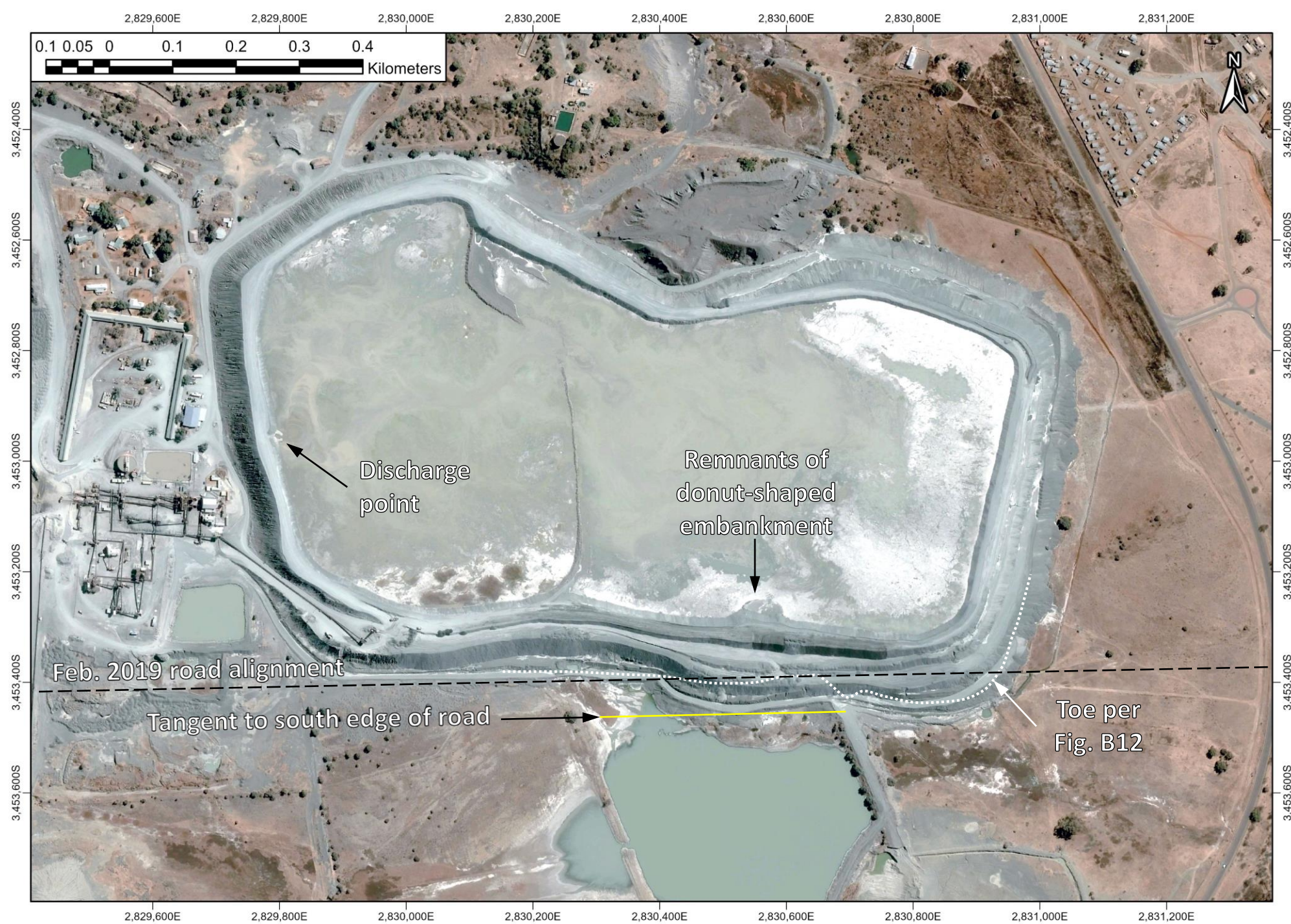
Figure B16: 2020-08-28 Pléiades 1 satellite image highlighting the separation between the February 2019 (Figure B10) and the current location of the southern edge of the southern access road. Remnants of the donut-shaped embankment built against the southern wall are visible.
