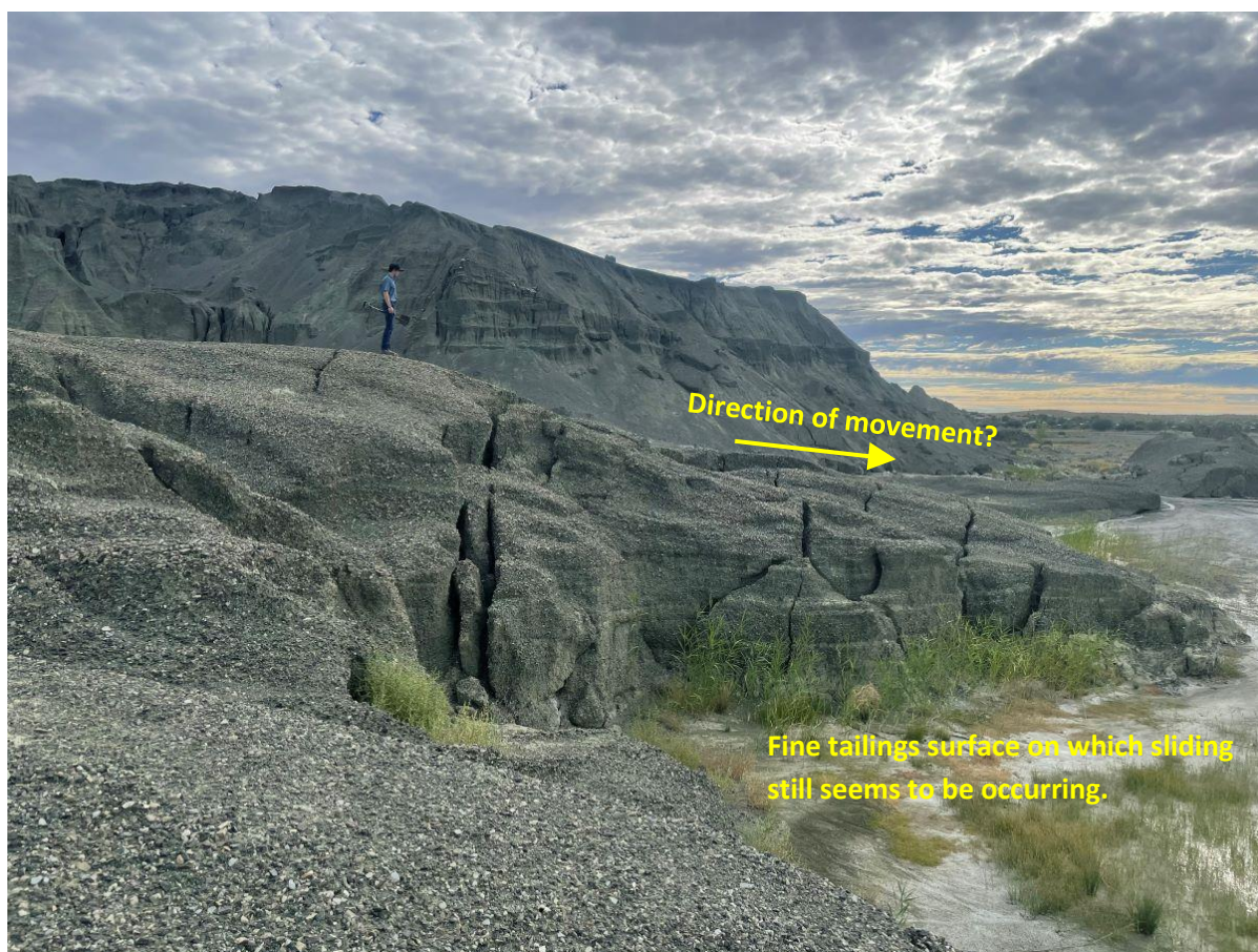
FIGURE 42 GRANULAR MATERIAL THAT REMAINED IN THE BREACH STILL SHOWING SIGNS OF MOVEMENT ON THE UNDERLYING LAYER OF TAILINGS. (LOCATION INDICATED IN FIGURE 41 ABOVE).
