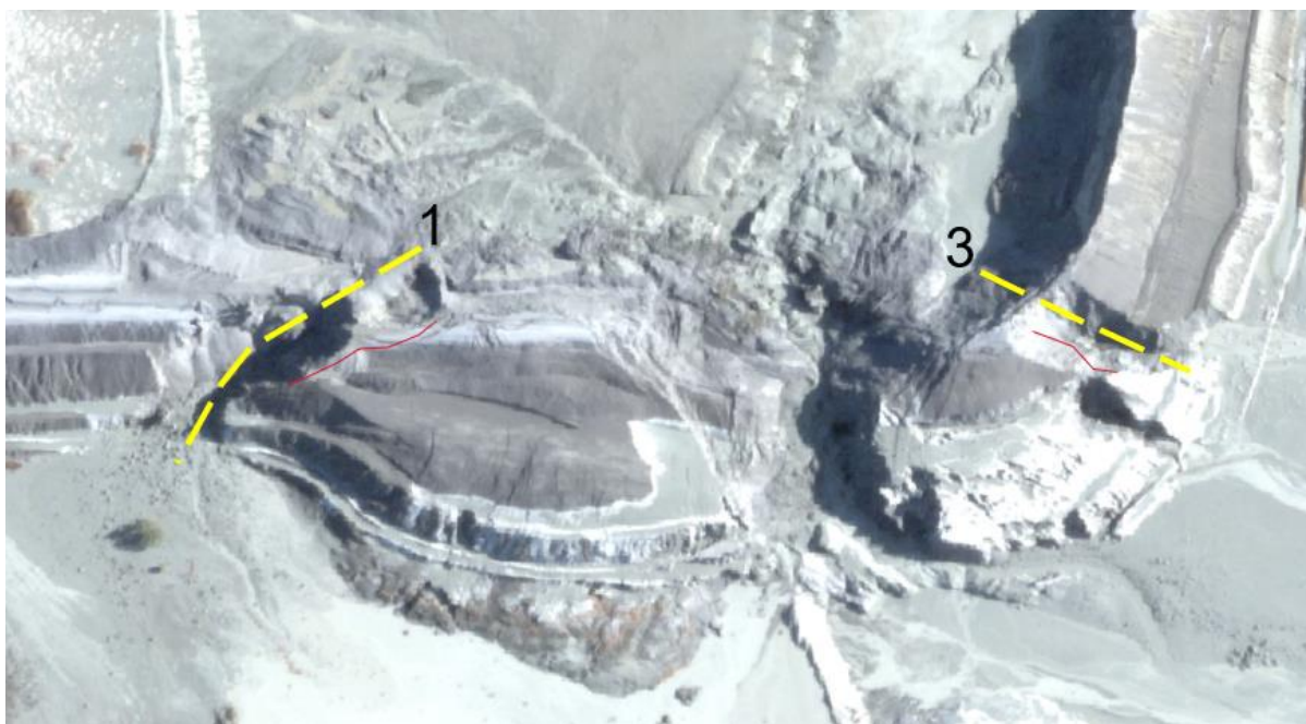
FIGURE 45 THE LOCATION OF CRACKS (IN RED) OBSERVED ON THE 24 SEPT 2020 SATELLITE IMAGE, SUPERIMPOSED ON THE FAILED SOUTHERN EMBANKMENT, SHOWS CLOSE CORRELATION WITH EROSION SCARS 1 & 3.
