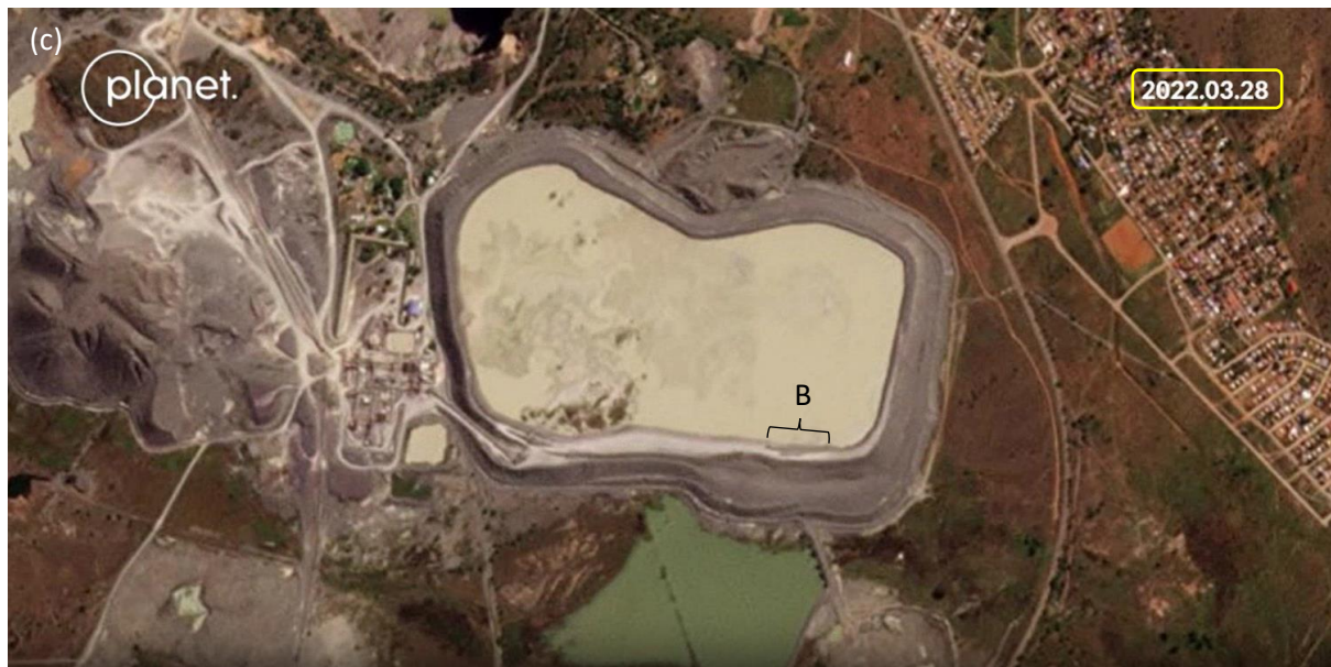
FIGURE 1 PLANETSCOPE IMAGES FROM MARCH 2022 SHOWING SIGNED OF INSTABILITY ALONG INTERNAL CREST EDGE OF DAM WALL.
