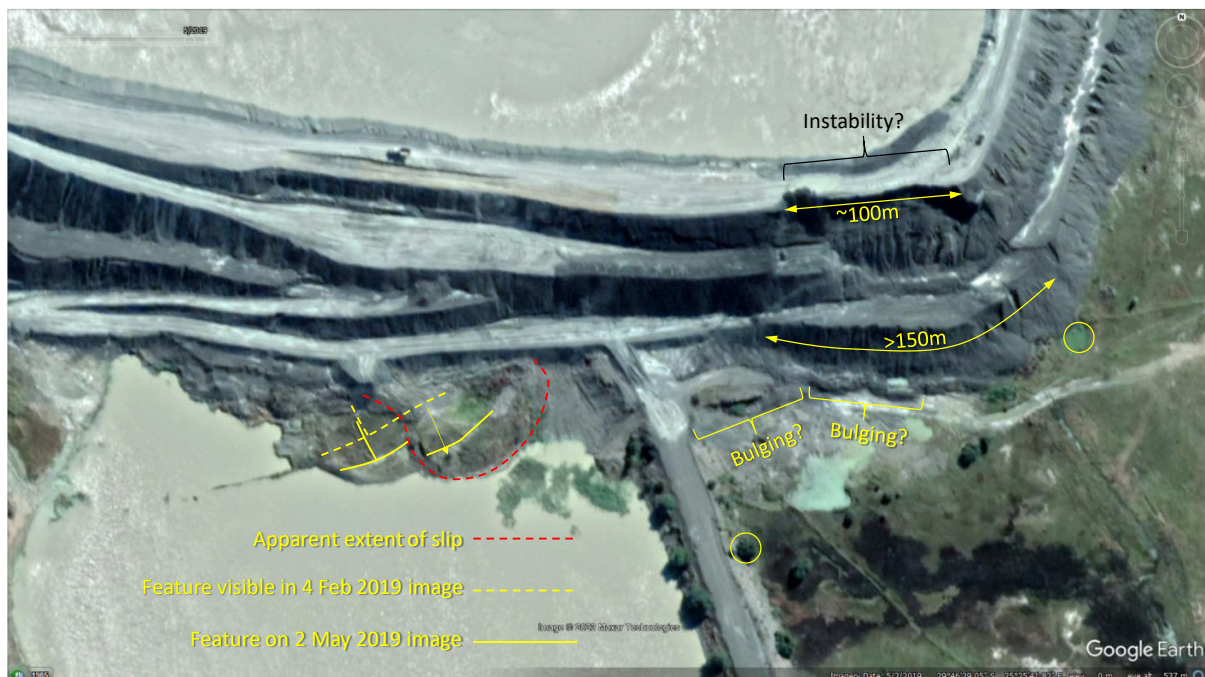
FIGURE 5 SOUTH-EASTERN CORNER OF THE JAGERSFONTEIN TAILINGS DAM FROM THE 2 MAY 2019 GOOGLE EARTH IMAGE SHOWING SIGNS OF INSTABILITY.
