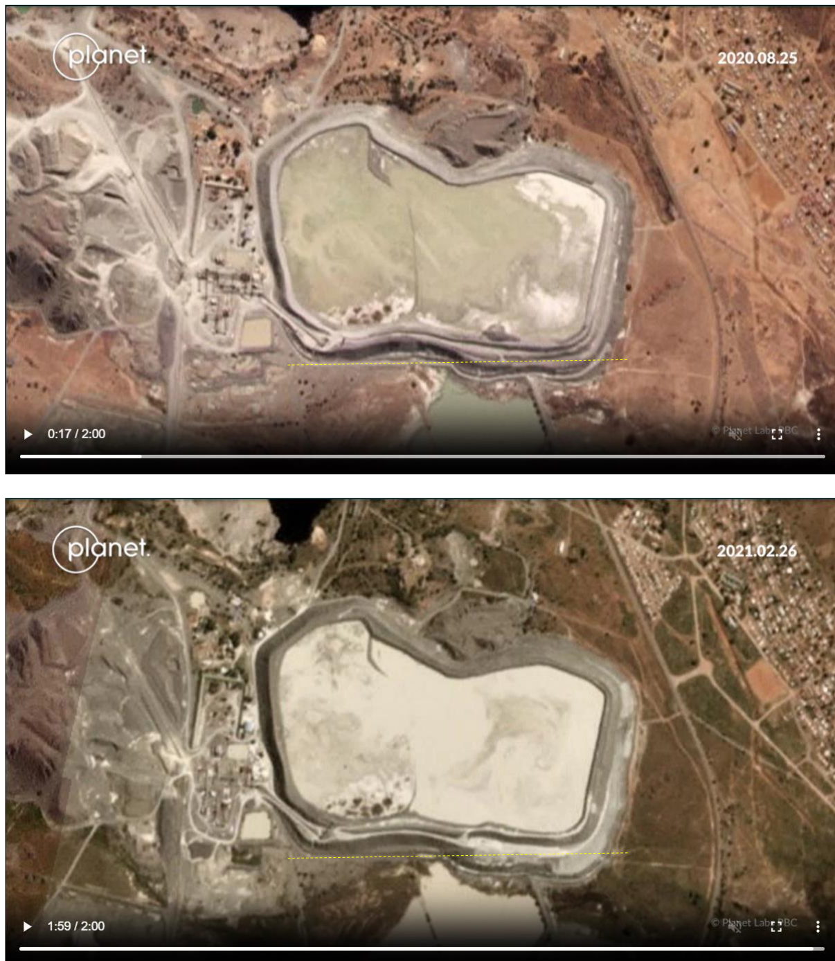
FIGURE 11 PLANETSCOPE IMAGING DATED (A) 2020/08/25 AND (B) 2021/02/26 SHOWING MORE DISPLACEMENT ALONG TOE OF THE SOUTHERN AND SOUTHEASTERN WALLS OF COMPARTMENT 2.
