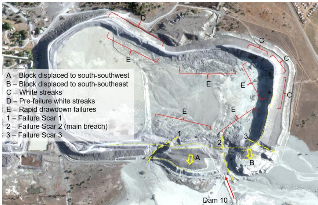
FIGURE 34 FEATURES ASSOCIATED WITH THE FAILURE EVENT. IMAGE FROM 12 SEPTEMBER 2022.
