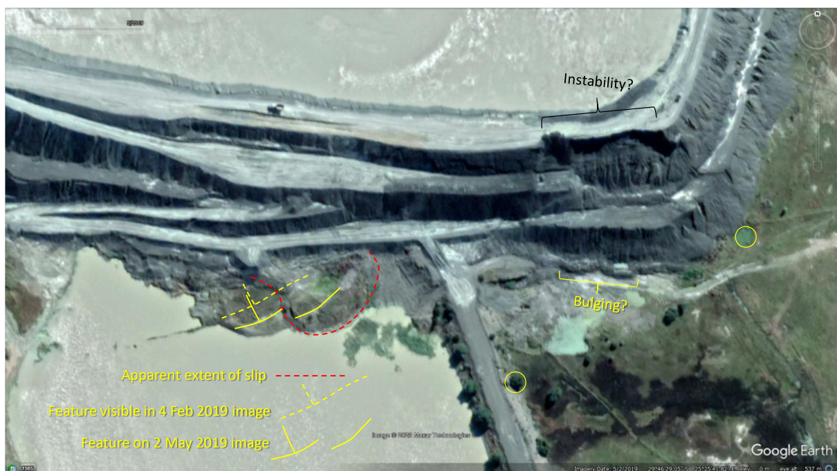
FIGURE 7 GOOGLE EARTH IMAGERY DATED (A) 2019/02/04 AND (B) 2019/05/02, WITH THE LATTER SHOWING SIGNS OF INSTABILITY IN THE SOUTHEASTERN CORNER OF THE DAM.
