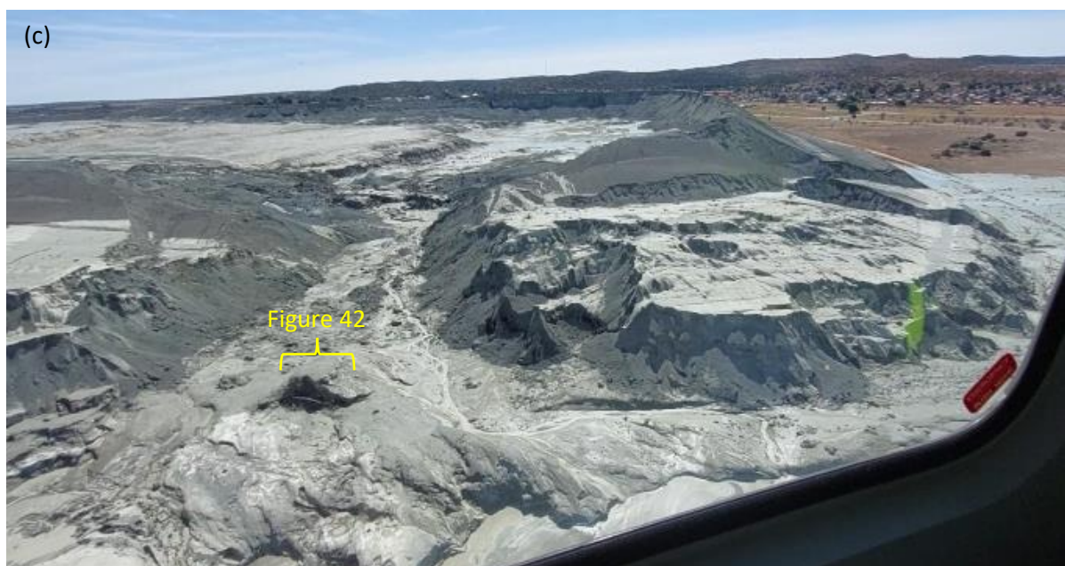
FIGURE 41 THE BREACH FLOOR COMPRISES A LAYER OF CONSOLIDATED TAILINGS THAT RESISTED EROSION DURING THE FAILURE. (A) LOOKING DOWN TOWARDS THE BREACH FROM THE EASTERN SIDE OF THE BREACH. (B) LOOKING SOUTH ALONG THE WESTERN SIDE OF THE BREACH. (C) TAKEN FROM HELICOPTER ON 12 SEPTEMBER 2022 SHOWING EMBANKMENT UNDERLAIN BY CONSOLIDATED TAILINGS.
