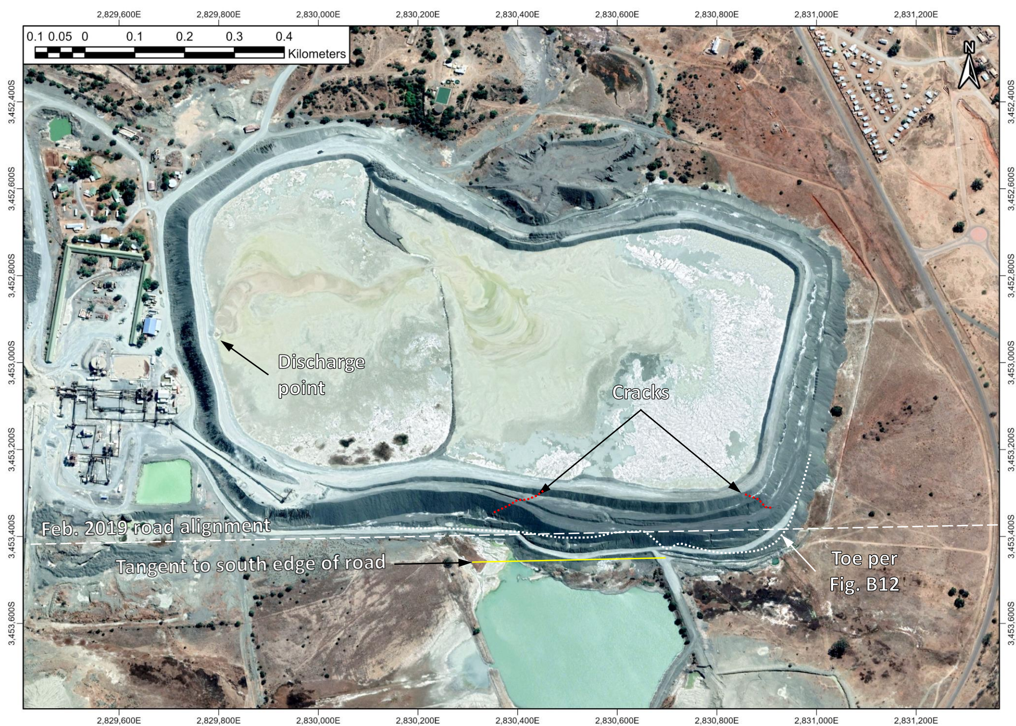
Figure B17: 2020-09-24 WorldView 2 satellite image highlighting the separation between the February 2019 (Figure B10) and the current location of the southern edge of the southern access road. Cracks visible in the southern wall are also indicated. Note: Cracks can be better appreciated by viewing the image in Google Earth Pro.
