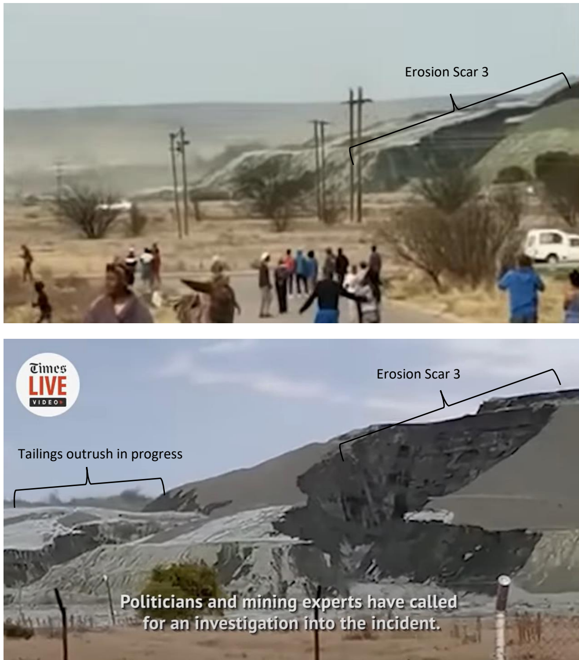
FIGURE 44 SCAR 3 ALREADY DEVELOPED AS THE OUTFRUSH OF FINE TAILINGS FROM THE DAM WAS OCCURRING THROUGH THE MAIN BREACH. (SOURCE: HTTPS://WWW.YOUTUBE.COM/WATCH?V= ND_LoNoj8Y ).
