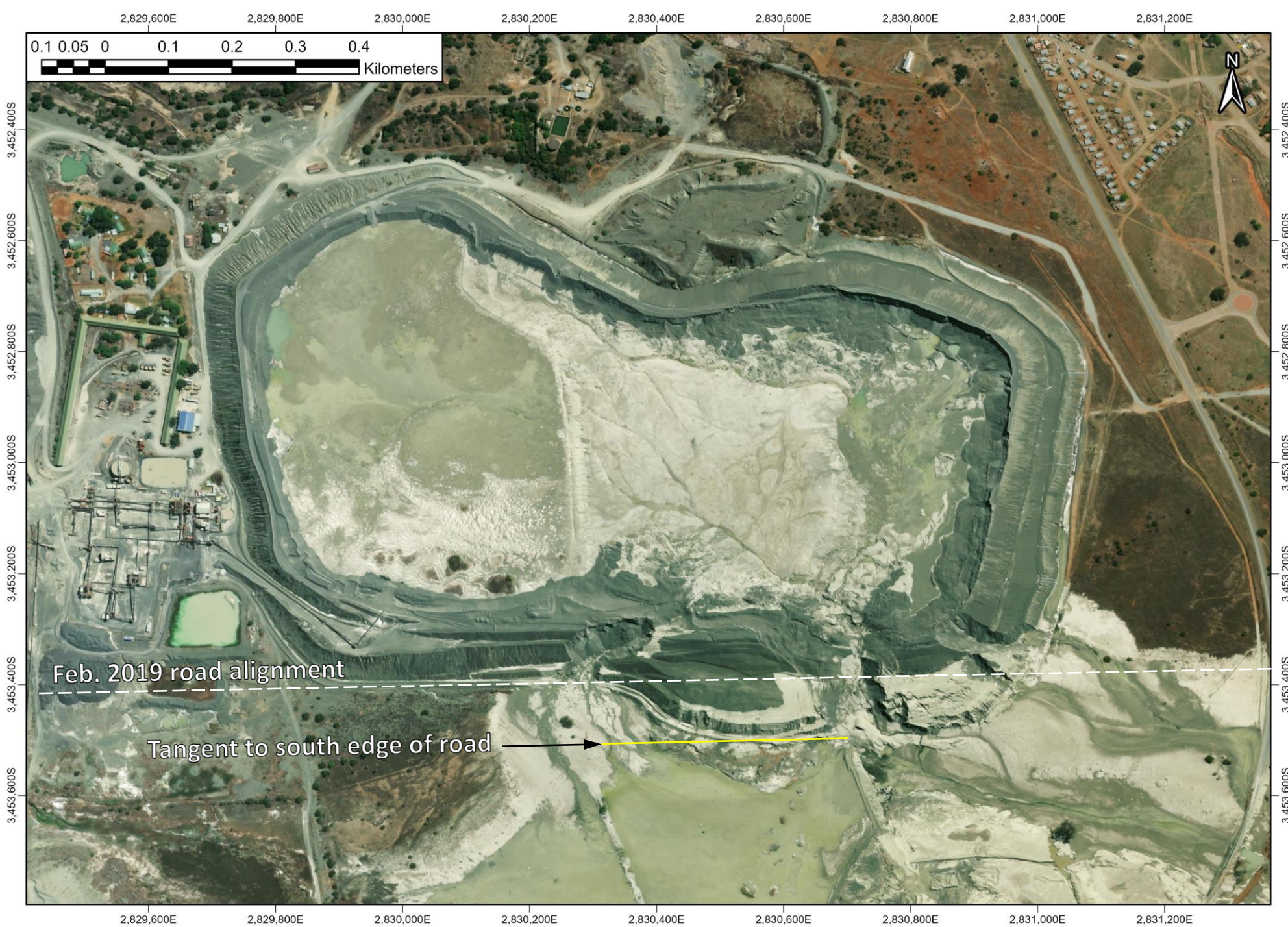
Figure B24: 2022-09-24 WorldView 2 satellite image highlighting the separation between the February 2019 (Figure B10) and the current location of the southern edge of the southern access road.
