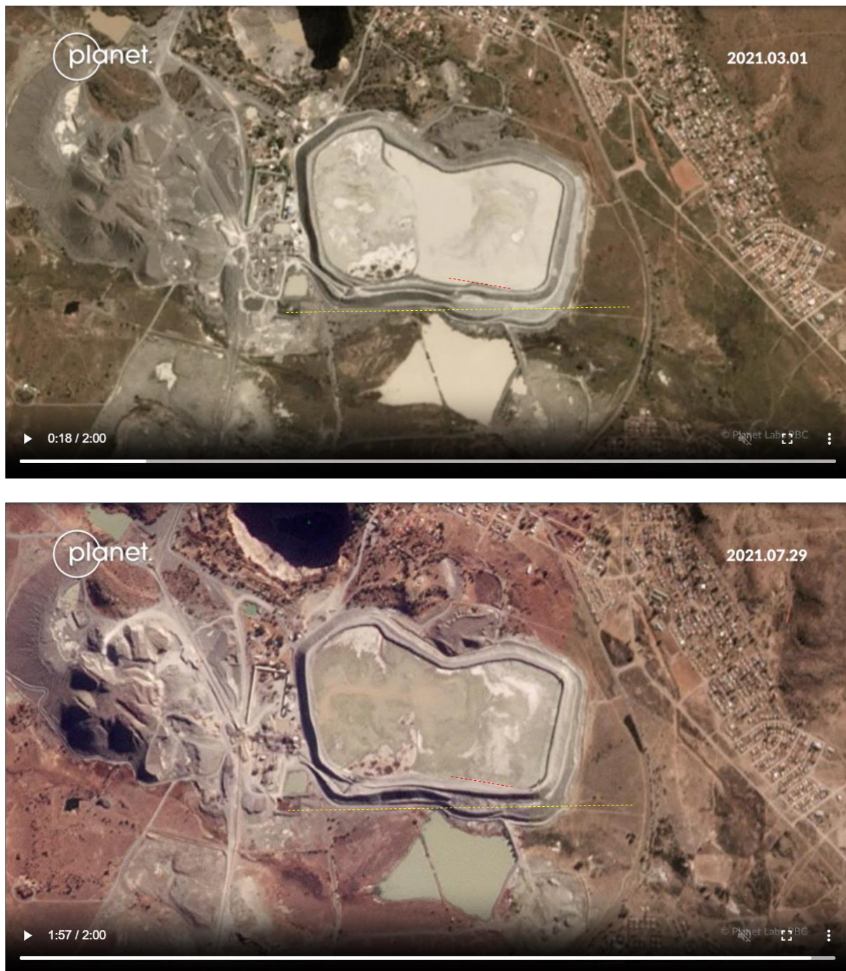
FIGURE 12 PLANETSCOPE IMAGING DATED (A) 2021/03/01 AND (B) 2021/07/29 SHOWING NO VISIBLE SOUTHWARDS MOVEMENT ALONG SOUTHERN TOE OF COMPARTMENT 2, BUT WALL RAISING EVIDENT (DOTTED RED LINE).
