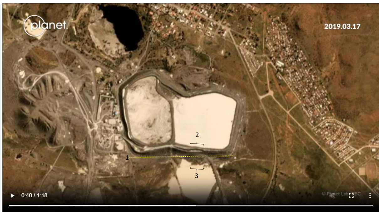
FIGURE 4 PLANETSCOPE SATELLITE IMAGES TAKEN ON 2019/03/13 AND 2022/03/17 SHOWING FURTHER SIGNS OF SLOPE INSTABILITY ALONG THE SOUTHERN WALL OF COMPARTMENT 2.
